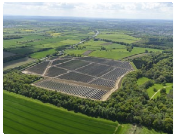
Eynsham solar farm, Oxfordshire
