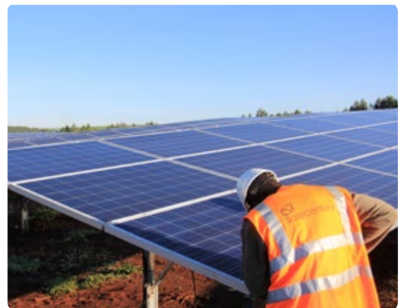
Kenya's largest solar farm
