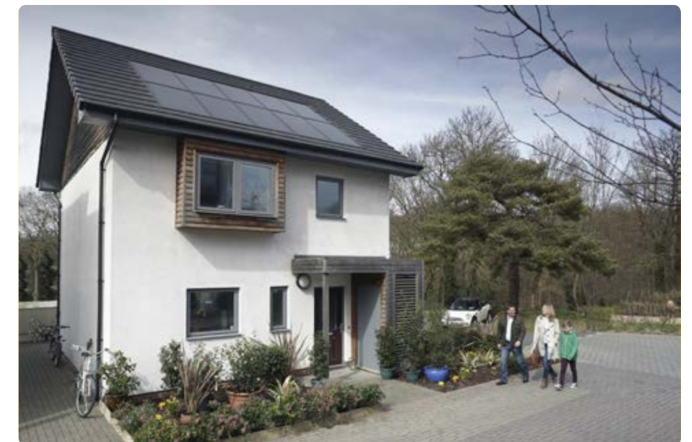
New product Sunstation launched and installed
